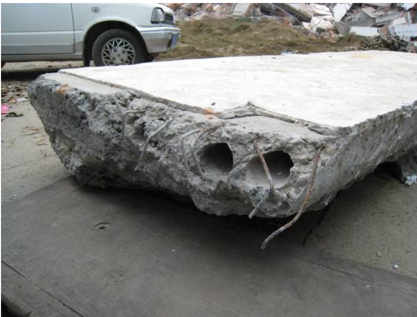
Photo2: Prefabricated floor slab referred in Photo 1
