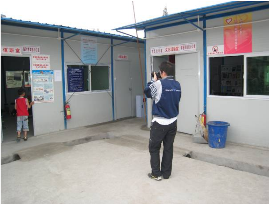
Photo 7 and 8: Temporary shelters in Dujiangyan City. It has drainage system, learning room, playing room, common kitchen, temporary clinic, and bathroom.
