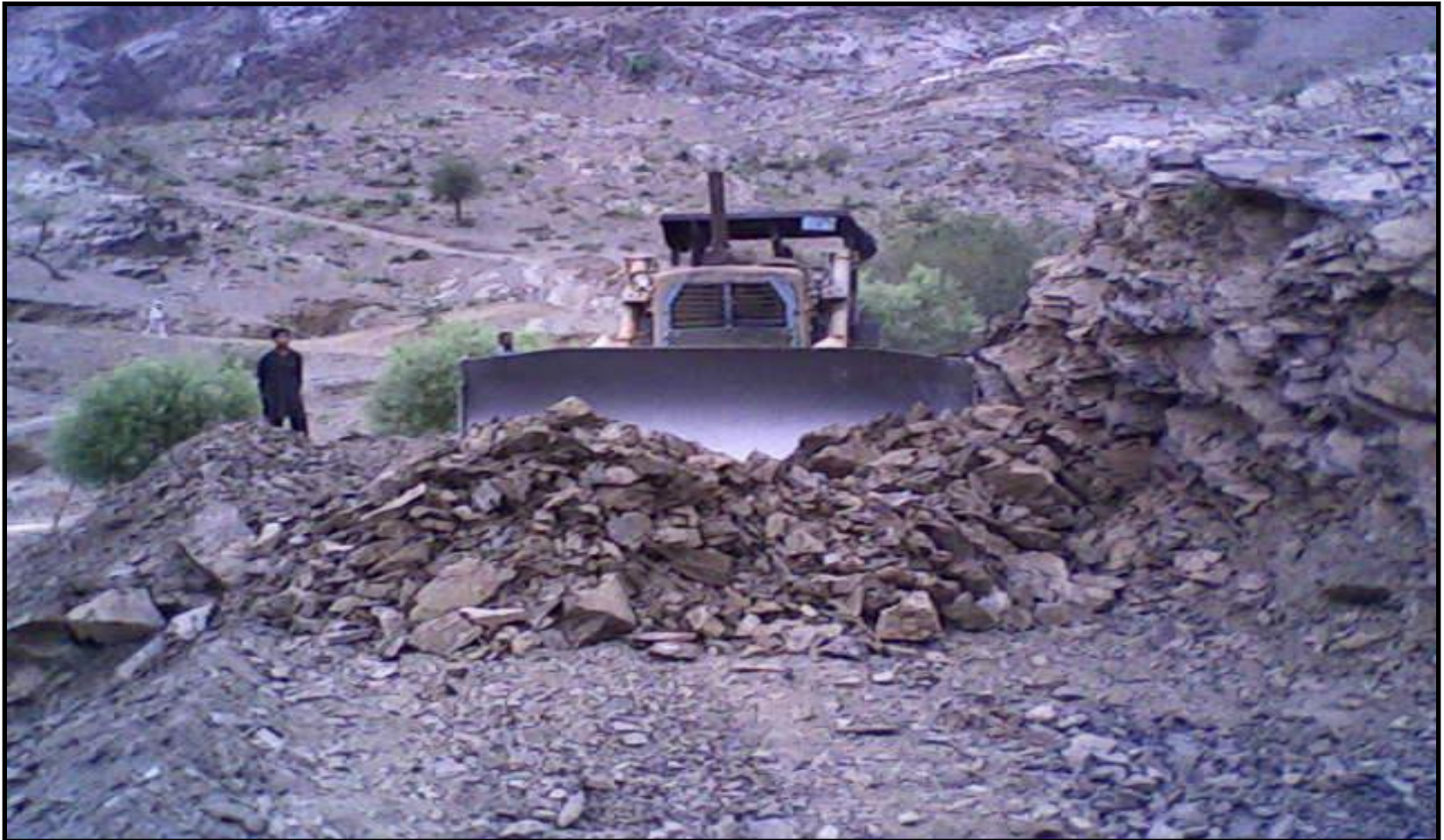
Shingle Road construction
