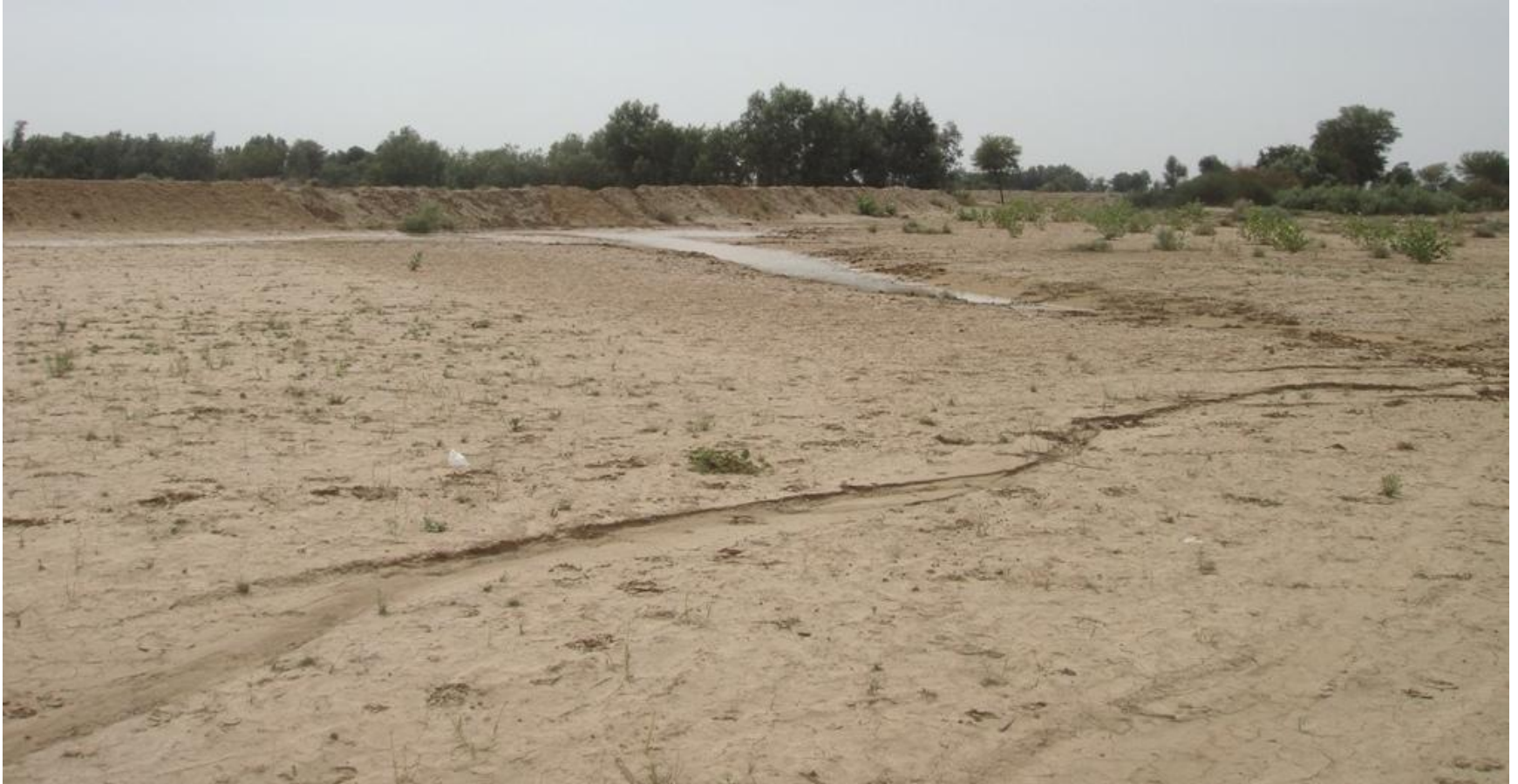
Earthen controlling structure – situation before the spate flood Source: Karim Nawaz
