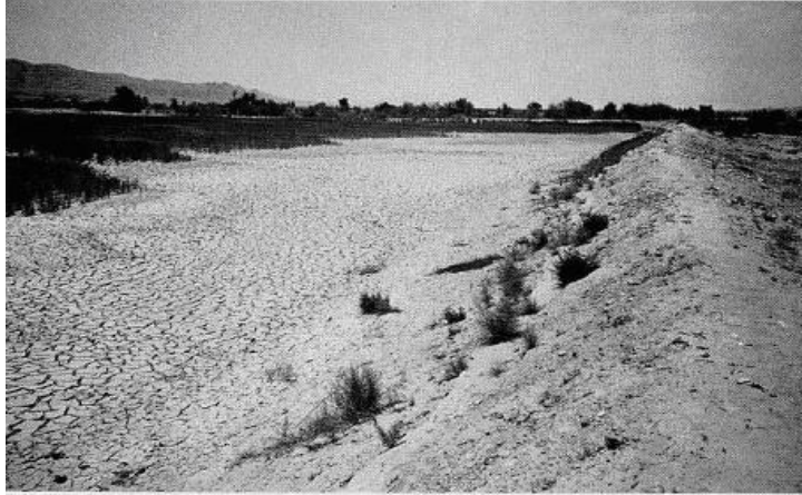
Bund made from local earth serving as a “receptacle” (“retention basin”, “compounding basin”) for water and soil
