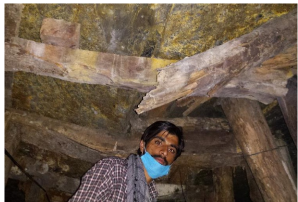
Plate 14: Timber support provided at roof has been broken due to pressure.
