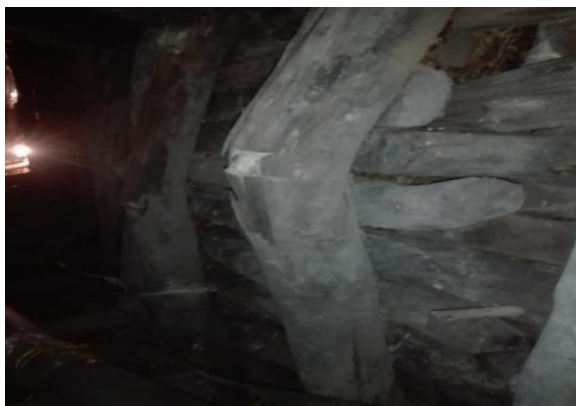
Plate 13: Timber bended due to weathering and ressure
