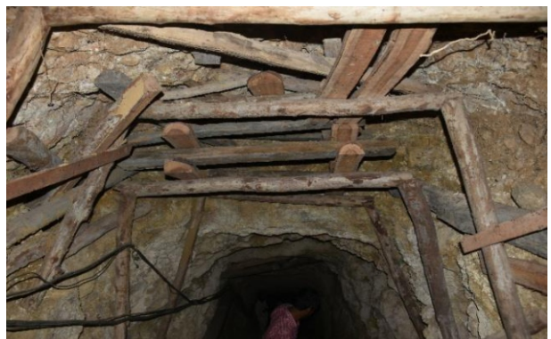
Plate 9. Poor roof supporting system in coal mines.
