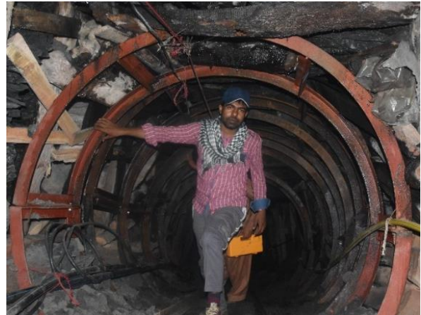
Plate 11. Iron horse shoe shaped support in coal mine no.5 to support the shale
