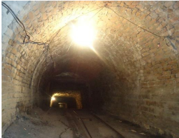
Plate 10. Brick wall in coal mines to support the shale.
