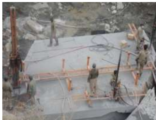
Fig. 7. Line drilling for filling of cracking powder (Rehman, 2010)
